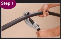
Unroll pipe into trench or on the ground and cut to desired length – plus one foot. Cutting up to 1" can be done with a large tubing cutter. For  $1\frac{1}{4}$ " – 2" sizes, a reciprocating saw is recommended.
