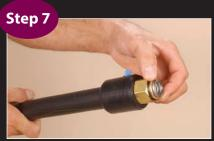
Remove adapter and split rings from fitting. Attach adapter to equipment. Slip coupling and nut over end of pipe all the way to expose first corrugations of pipe. Insert split rings into first corrugation as shown.
