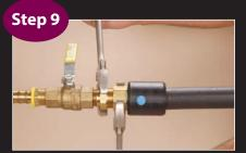
Thread the nut onto adapter previously installed on the equipment. Using appropriate wrenches, hold adapter and tighten nut to proper torque specified. <u>Do not overtighten</u> <u>or use any thread sealants on this connection.</u> <u>This is a metal-to-metal seat and will not</u> <u>seal if pipe dope or thread sealants are used.</u> <u>Sealants are to be used on the NPT connection</u> <u>to the equipment only!</u>
