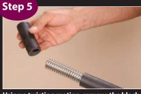
Using a twisting motion, remove the black sleeve and yellow jacket from the pipe. It may be necessary to cut sleeve longitudinally and peel off on larger sizes. <u>Inspect stainless pipe</u> for scoring from the tubing cutter.
