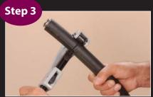
Using the appropriate tubing cutter with TracPipe #FGP-E-5272 Cutting Wheel, score the black sleeve approximately half of the way through. Use extreme care not to cut down to the stainless corrugated pipe. No more than two turns in on the cutter is sufficient. Inspect tube for scoring from the tubing cutter.
