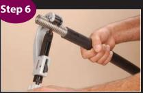
Using the tubing cutter, trim corrugated pipe to strip length specified on the Strip Length Chart shown above. Cut slowly in the root of the corrugation in the same manner you would cut copper tubing. Inspect end of pipe for a clean cut without tears in corrugation.
