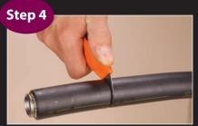
Carefully, finish cutting through the sleeve down to the stainless corrugated pipe using a sharp utility knife.
